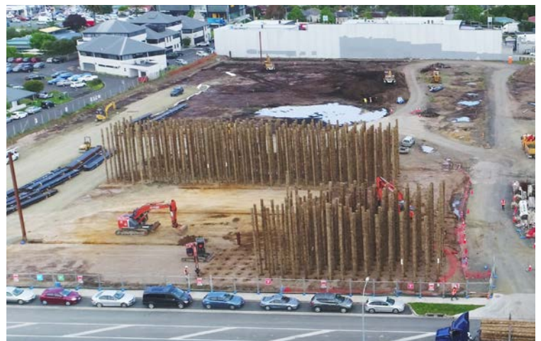
Photos courtesy of Markovina Pile Driving
